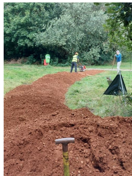
An idea of the amount of hard-core required
