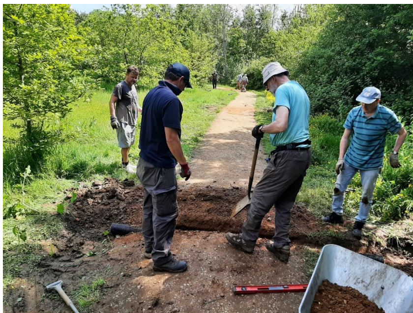
Installing a drain across the path
